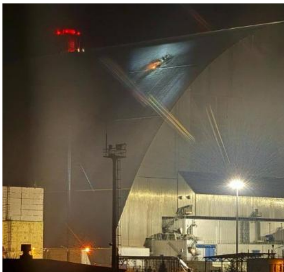
Fig. 1. Fire at the Chernobyl NPP reactor in 2025
